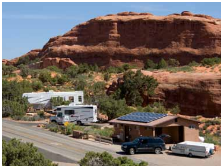
Solar panels cover the roof of a comfort station at the Devils Garden Campground.
